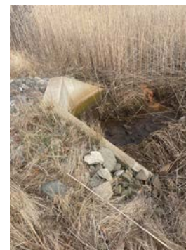
Photo #18 -- Culvert at RV S side
