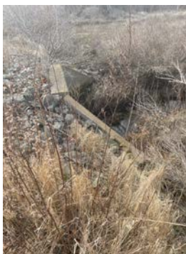
Photo #17 -- Culvert at RV N side
