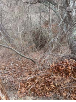
Photo #1 -- Possible culvert opening
