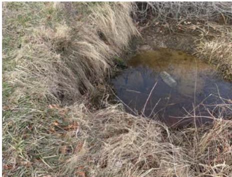
Photo #15 -- Culvert Rv to CC low tide E side
