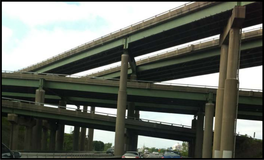
Figure 1. Connecting ramps for the I-90 bridge across the Hudson River. Photo: G. Stahl, Albany, NY, 2012.
